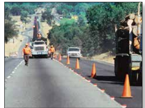
Super TRPMs retain the original lane line location to aid in re-striping
